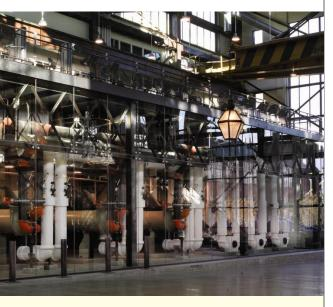
At this retailer's headquarters, a 3,400-ton central plant was constructed and installed with three chillers and all associated equipment. The new and improved system provides more efficient operation and dramatic energy cost savings to the entire headquarters campus.
